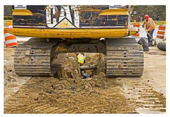
"Trench construction, safety: Caterpillar 3128 crawler mounted backhoe straddles trench for underground pipe. Worker in trench is fine grading/cleaning trench with shovel. Workers standing in 8ft deep trench have no support against sidewall collapse. Safety and laws require the trench walls to be supported or sloped back at depths greater than 5ft."
