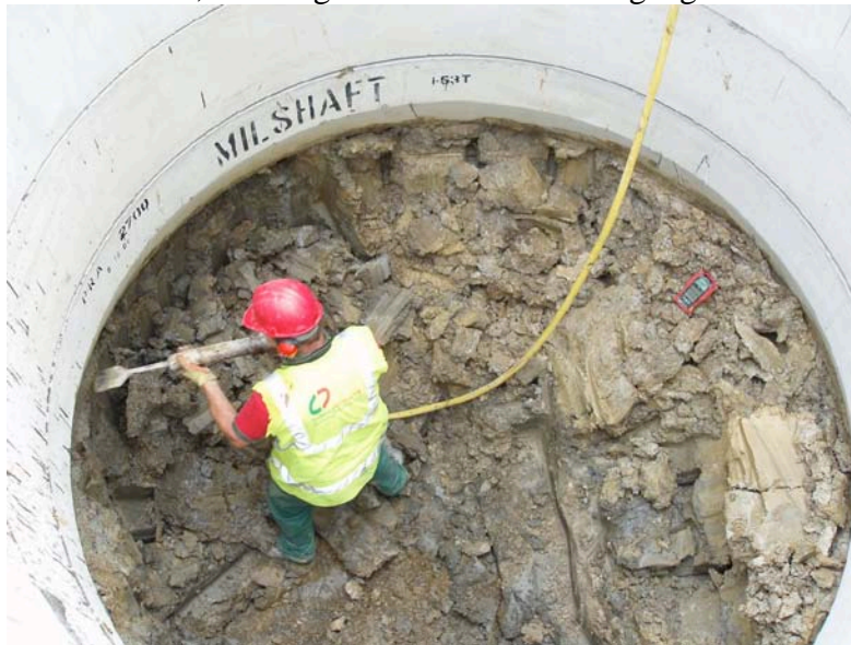
Hand excavation at the cutting shoe, allowing the caisson to sink in a controlled way
