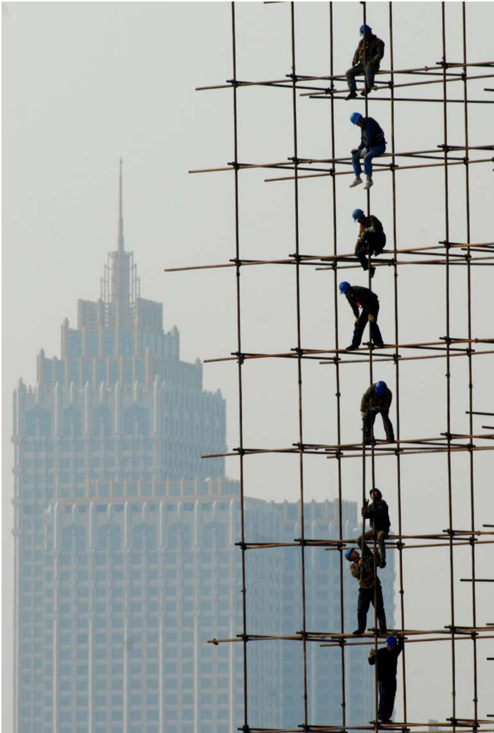
Workers erect scaffolding in Shenyang in NE China (From The Guardian 24 March 2009)
