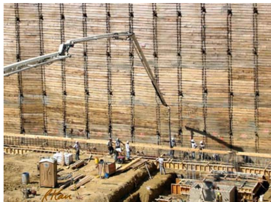
(Photo: Robert Carr, http://myconstructionphotos.smugmug.com ) Concrete pump providing concrete in a deep excavation
