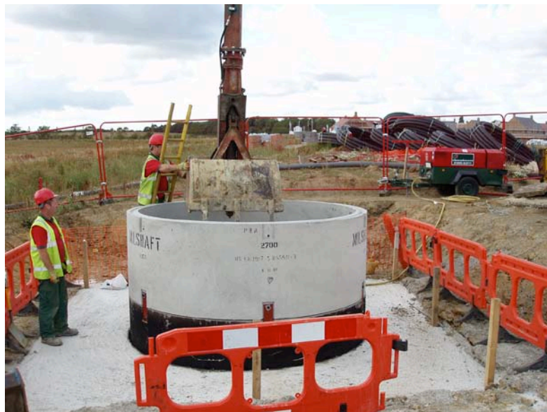
An actual installation, showing bulk excavation using a grab on an excavator
